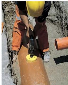
**1** Drill the pipe squarely with a cylindrical saw  $\varnothing = 152\text{mm}$  (6").
