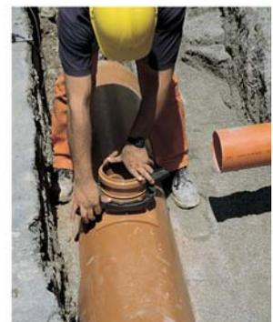
**3** Screw the ring nut with the appropriate clip until the blocking of the obtained branch.
